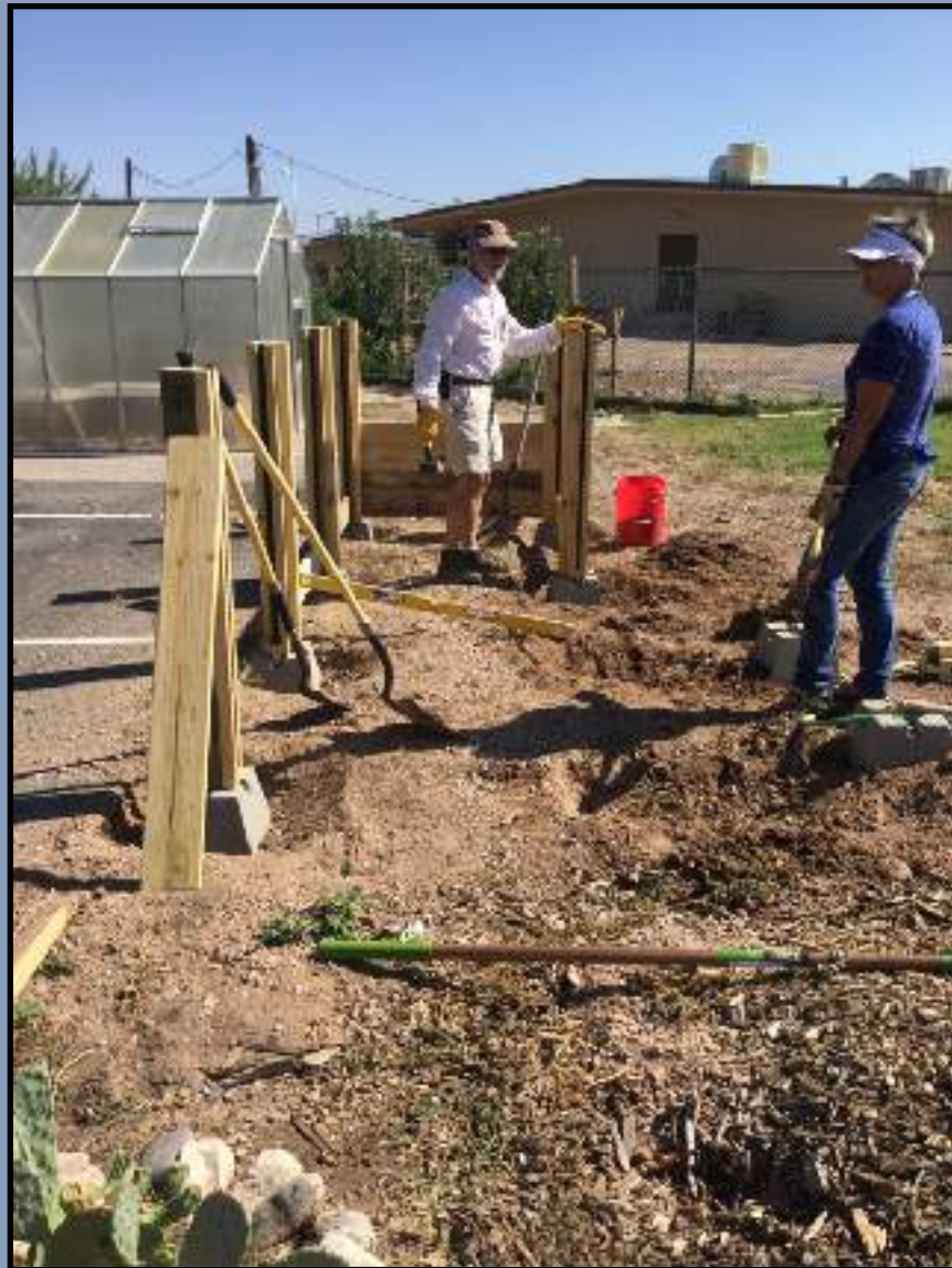
4. Setting, leveling and squaring of side support posts
